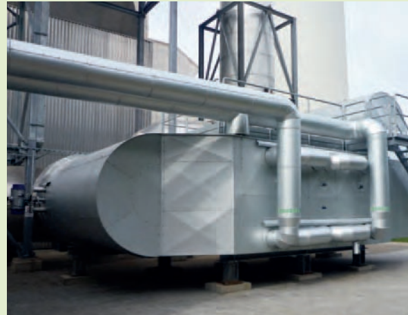
A waste heat boiler installed at Weiherhammer, Germany.
